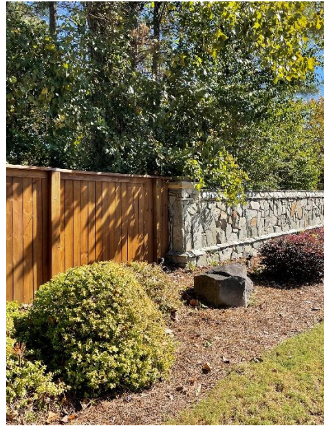
New Fence installed April/stained July
